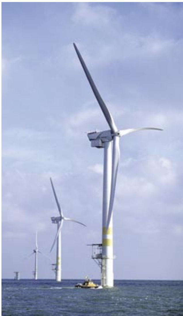
GE wind turbines installed in the Irish Sea.
