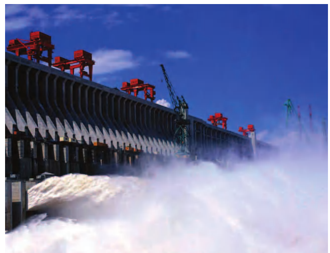
Three Gorges Dam, China
