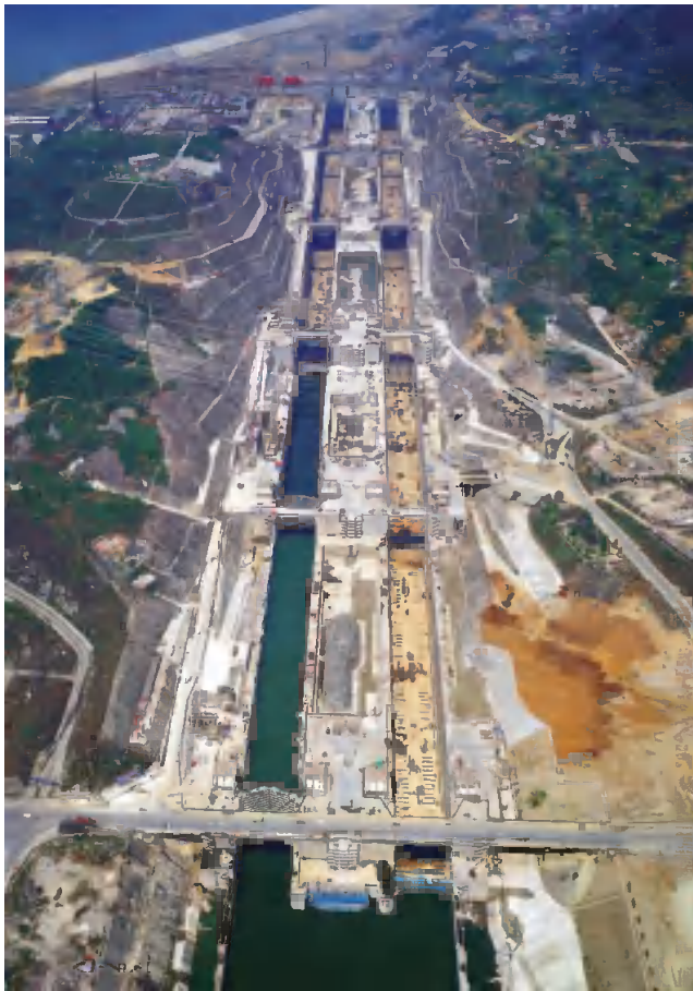
Three Gorges Dam, China
